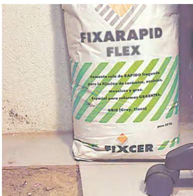
Urgent office repairs
