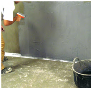
The 1st coat of HIDROFIX.
