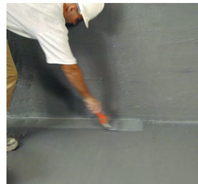
The 2nd coat of HIDROFIX.
