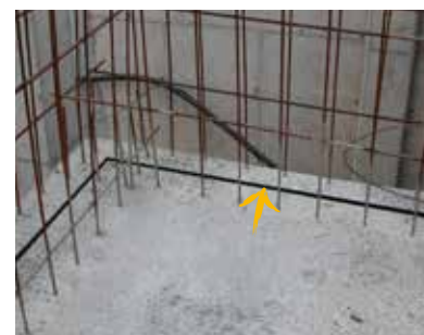
Application of FUGA-STOP 25 x 20 mm
