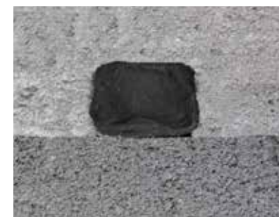
FUGA-STOP 25 x 20 mm once in place
