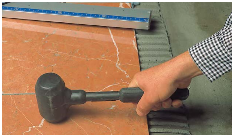
Pack the pieces solidly to ensure good bonding.
