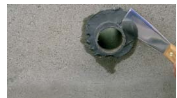
Smooth the entire surface.
