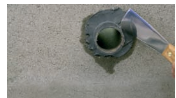
Smooth the entire surface.
