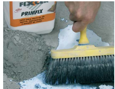
Bonding paste: PRIMFIX + pure Portland.
