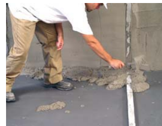
Spread uniformly between guides.
