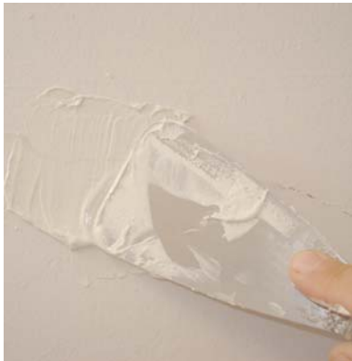
Fill and smooth all cracks and holes.
