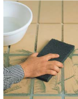
Use the FIX-BUCKET and the cleaning trowel.
