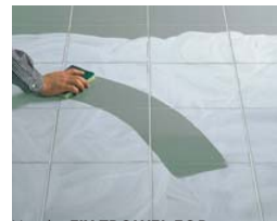
Use the FIX-TROWEL FOR CLEANING .
