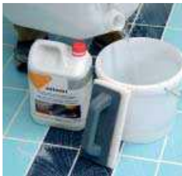
Do final cleaning after 7 days using one part GRESNET diluted with 10 parts water.
