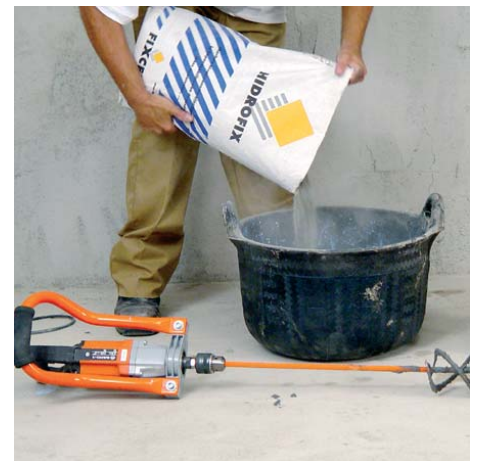
Mix HIDROFIX with water using a mixer.
