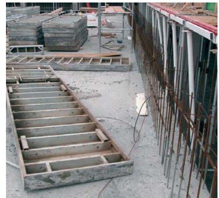
Pack the FUGA-STOP and pour concrete between the moulds.
