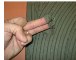
Check the adhesive is fresh.
