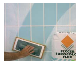
Seal 24 hours after laying tiles.
