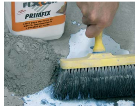
Bonding paste: PRIMFIX + pure Portland.
