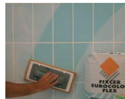
Grout after 24 hours have passed since laying.
