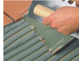
Use the double gluing method.
