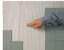
Make sure the cement is fresh.
